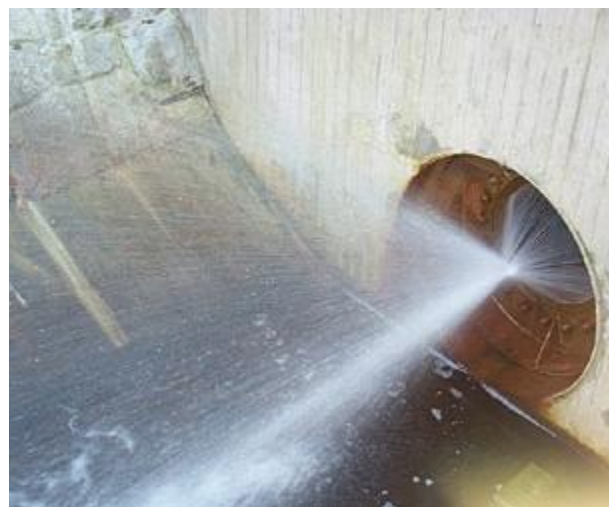
Figure 6: Concentric dissipation of energy directly downstream of a VAG Plunger Valve DN 800
